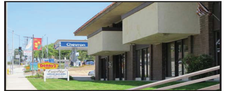
Canyon View Offices at 21308 Pathfinder Rd., Diamond Bar
